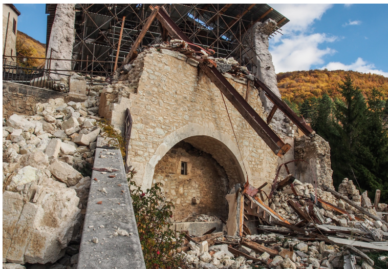
Unframed structure damaged by earthquake, Italy, 2017. Photo: Eisuke Nishikawa.
