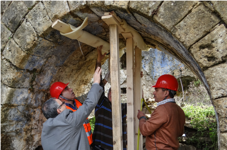
Emergency stabilisation in practice at a workshop in Shouf, Lebanon, 2014. Photo: ICCROM-ATHAR.
