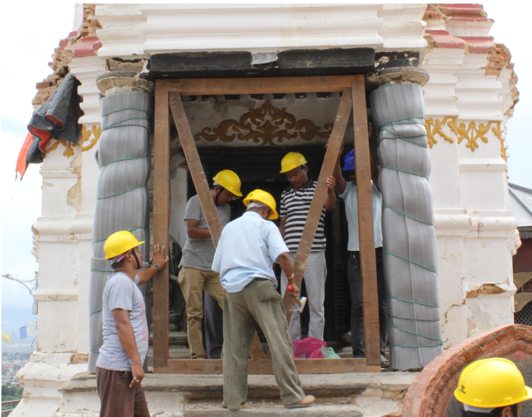
Emergency stabilisation of a temple in Kathmandu, Nepal, 2015. Photo: ICCROM.
