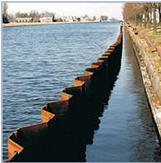
Figure 6.25 Use of piling for levee raise (courtesy Environment Agency)
