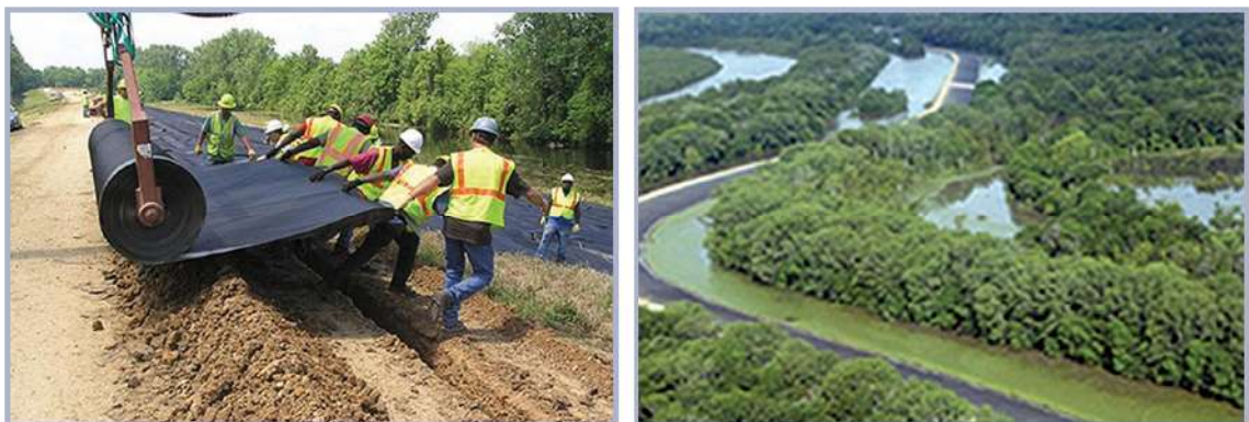
Figure 6.32 Use of plastic sheeting to prevent overtopping/overflow erosion, placing plastic sheeting on levee waterside (a) and finished placement (b) (courtesy USACE)
