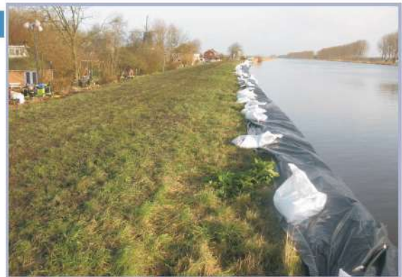
Figure 6.36 Use of impermeable sheeting to reduce infiltration (from DWR, 2010, and courtesy Henk van Hemert)
