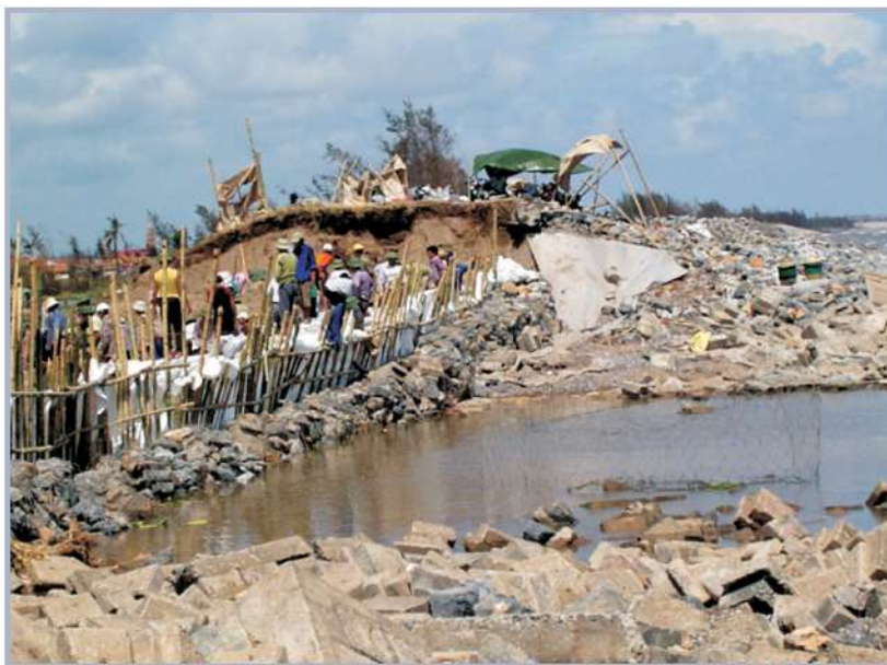
Figure 6.45 Emergency repair of coastal levee Nam Dinh, Vietnam after Storm no.7 (2005) (courtesy VNICZM project, Nam Dinh pilot office)
