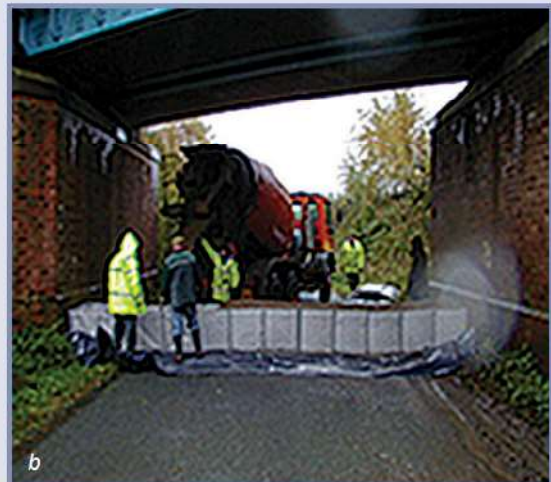
Figure 6.14 Levee breach in Gowdall (a) and temporary dam under construction on roadway under Drax railway line (b) (courtesy Environment Agency)
