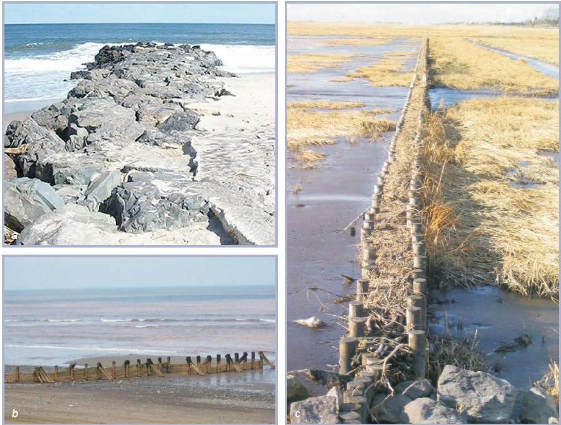
Figure 6.30 Examples of rock groyne (a), timber groyne (b), and earthfill groyne (c) (courtesy Wikimedia Commons)
