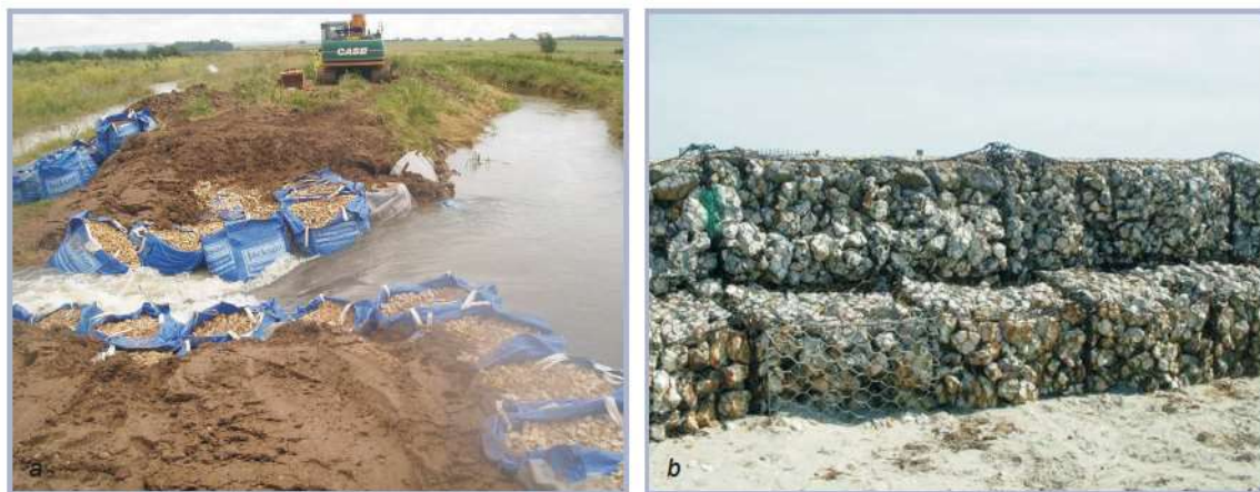
Figure 6.44 Response to levee breach, limiting breach growth using big bags (a) and gabions (b) (courtesy Environment Agency)
