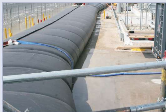
Figure 6.50 Water inflated barrier field setup (courtesy USACE)
