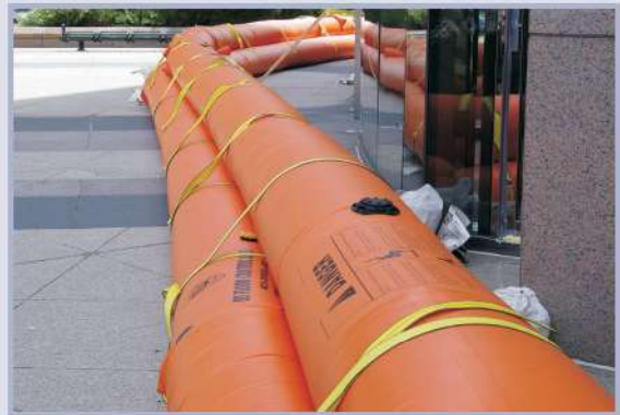
Figure 6.51 Tiger dam system implementation (courtesy USACE)
