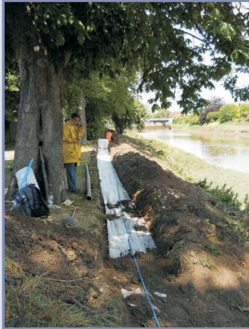
Figure 6.4 Fibre optic cable in geotextile fabric being laid in levee to measure ground strains at a pilot site (courtesy Victoria Bennett, RPI)
