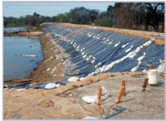
Figure 6.35 Use of impermeable sheeting to reduce infiltration over large area (a) and field application (b) (from DWR, 2010 and courtesy USACE)
