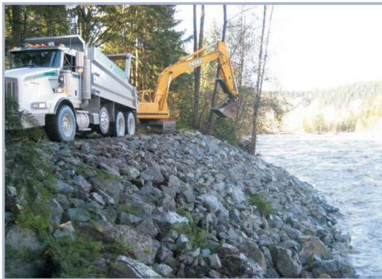
Figure 6.28 Construction of a rock revetment (courtesy USACE)
