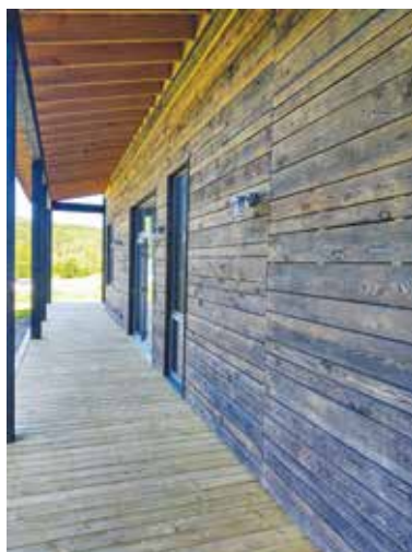
The Shou sugi ban siding.
