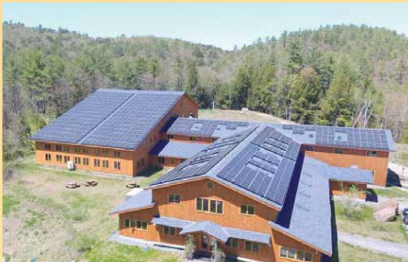
The 486.7kW rooftop solar array at W.S. Badger is expected to generate approximately 600,000 kWh of clean electricity per year which will cover 100% of Badger's electrical needs. Photos courtesy W.S. Badger.
