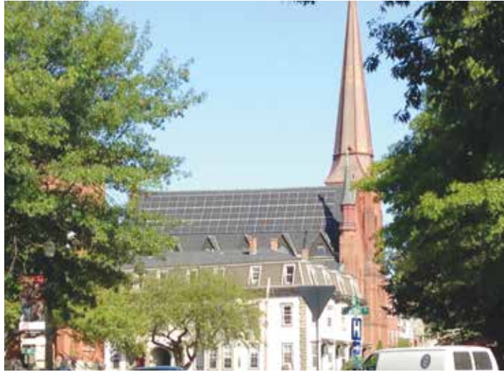
Paragon Digital Marketing renovated and moved operations to this vacant historic church in Keene, using CDFA financing to add 34 kW of solar. The company also installed air-source heat pumps, LED lighting and made significant improvements in air sealing and insulation. Photo: Scott Maslansky.
