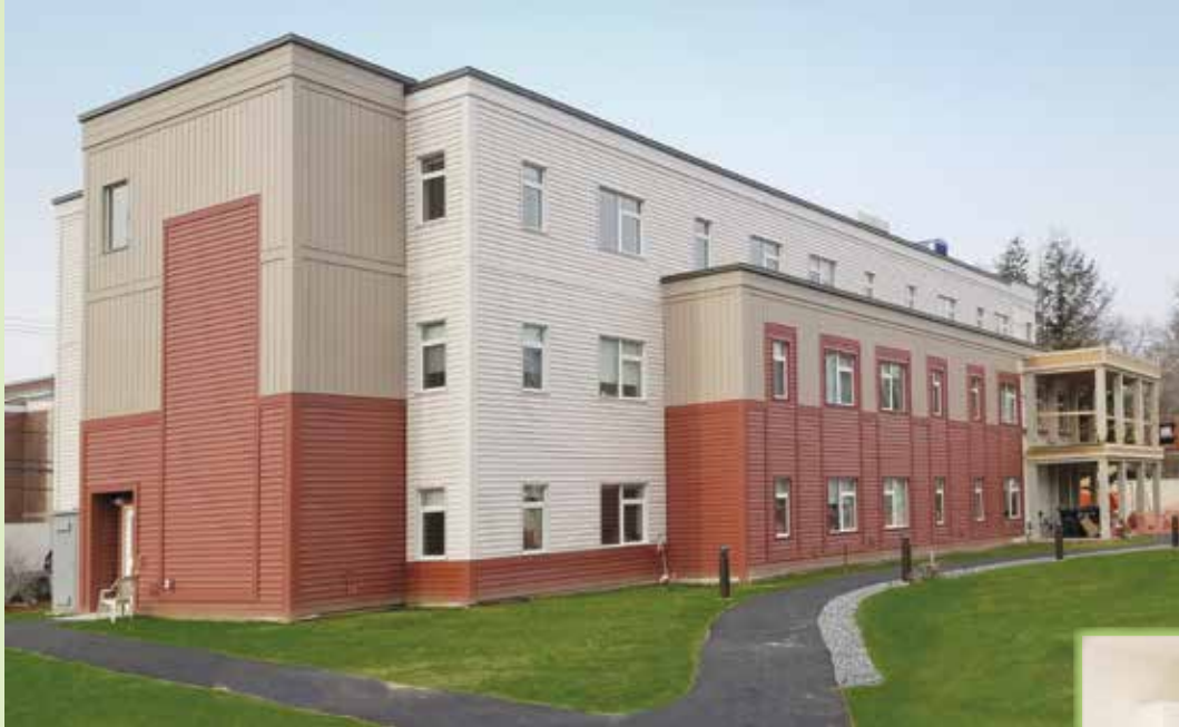
Summer Park Residences in Hanover, NH, is a Passive House certified, affordable housing building for seniors and those with disabilities. Twenty-four units are open with eighteen more under construction. Photos: Banwell Architects.
