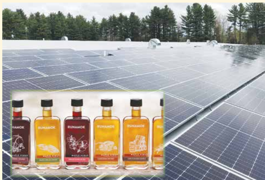
In March 2019, Norwich Solar Technologies installed a 150 kW-AC solar system powering Runamok Maple's manufacturing processes in Fairfax, VT. Runamok Maple is a premium, organic maple syrup producer. Courtesy photos.
