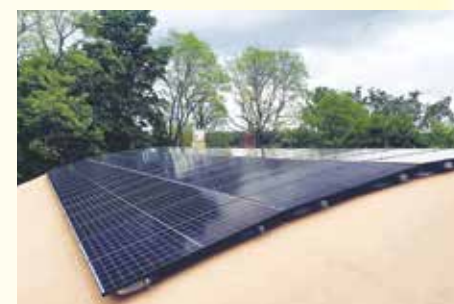
Top: Claremont MakerSpace has a 57.9-kW solar system, with savings of $7,100/yr., that offset approximately 28,732 lbs of CO 2 emissions per year. Claremont Soup Kitchen has a 27-kW solar, saving nearly $3200/year. The solar panels follows the curve of the roof. Photos: ReVision Energy.
